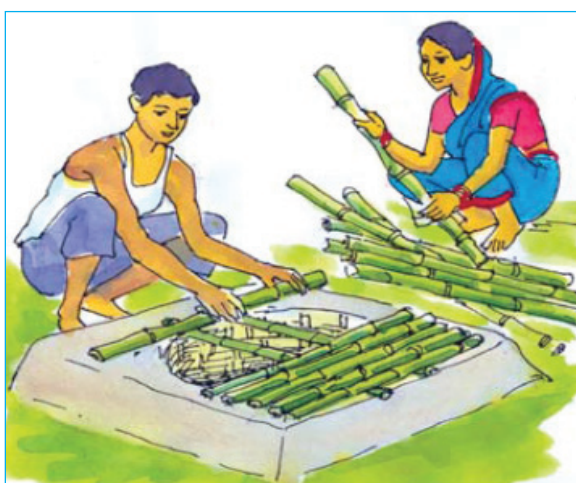
Construction of a platform floor on the pit
