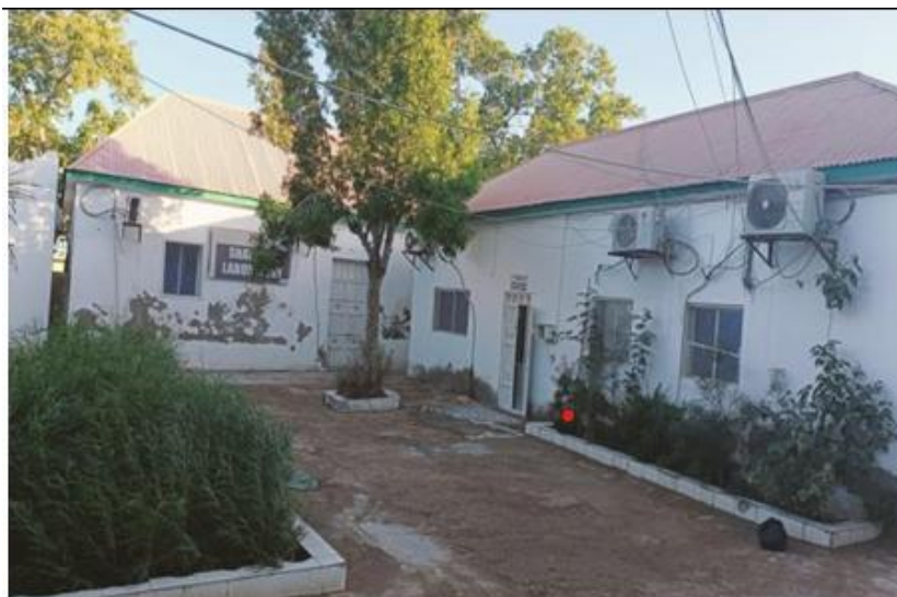
Figure 9 Existing Facilities of Bosaso Hospital
