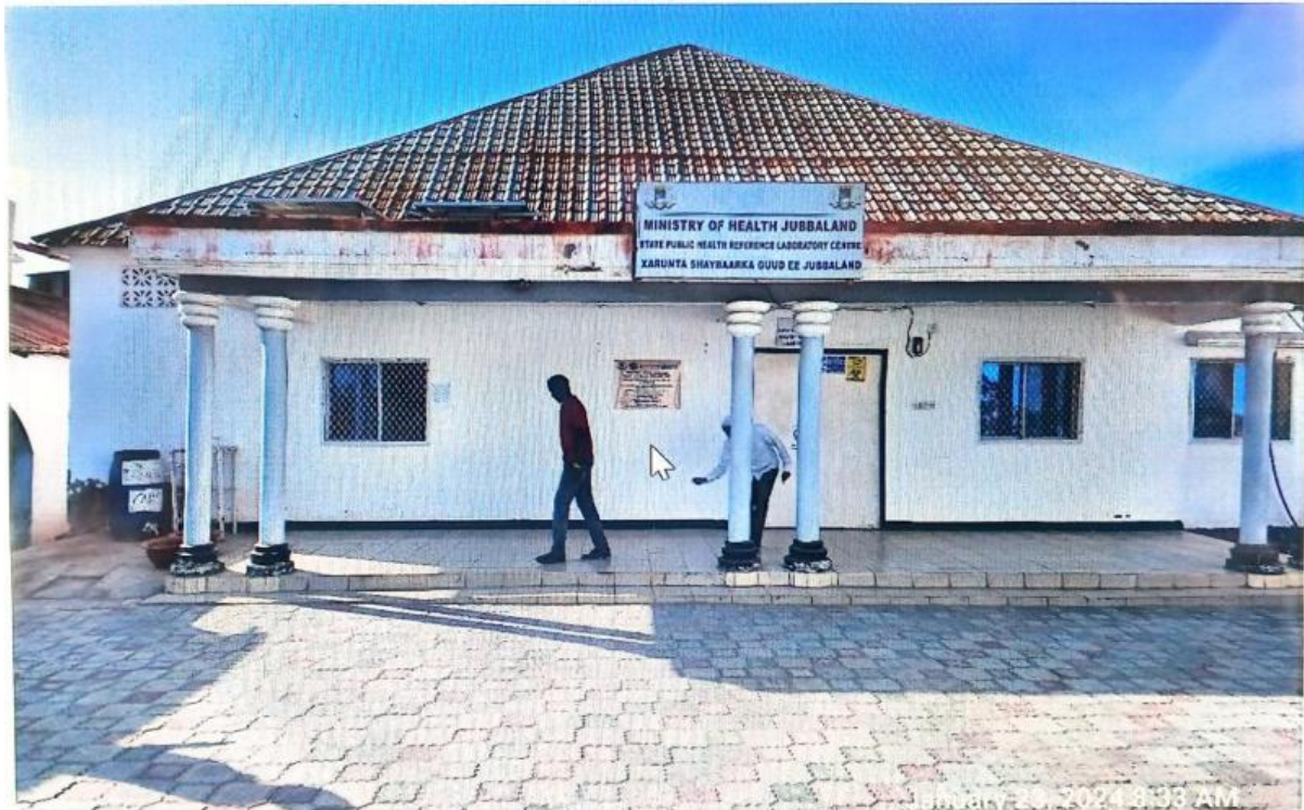
Figure 10 Existing Facility at Kismayo Hospital
