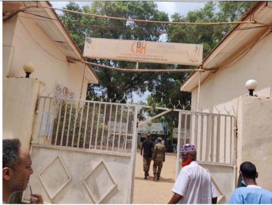
Figure 9 View of the existing building
